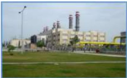
North Giza P.P (2250 MW) 1250 MW Completed
