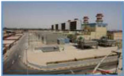
6 th October P.P (600 MW) 600 MW Completed totally
