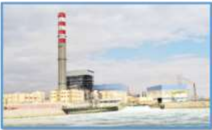
SUEZ P.P (650 MW) 250 MW Completed
