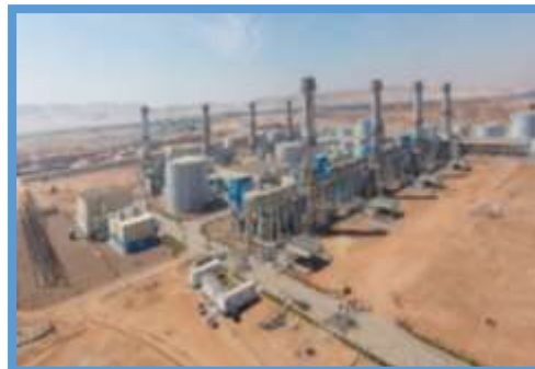
Assuit P.P adding 500 MW (Total capacity : 1500 MW)
