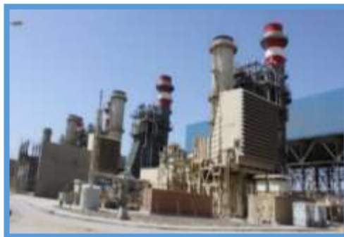
Shabab P.P adding 500 MW (Total capacity : 1500 MW)
