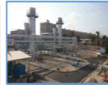
Port Said PP 84 MW
