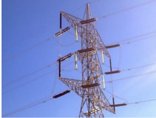
Figure 0-8 Example of the Double Circuit Tower to be used
