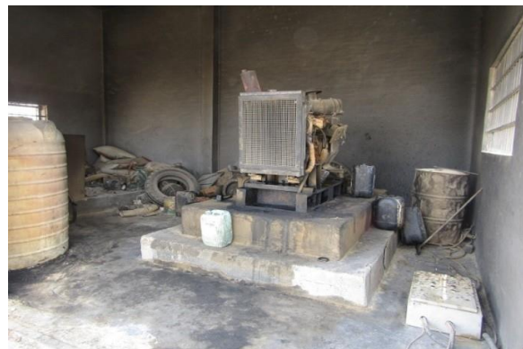
Figure 5-35: Diesel-based electricity generator
